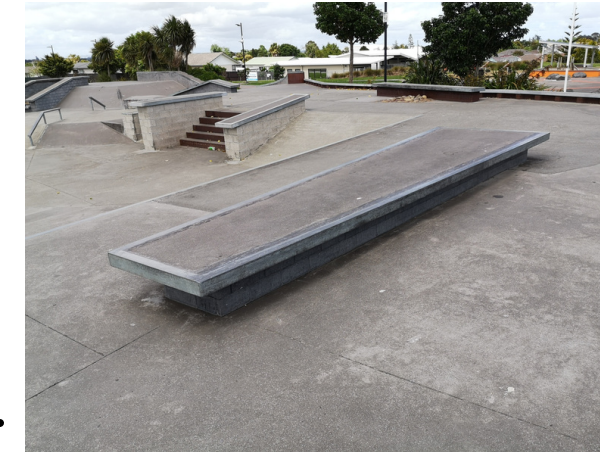
5000mm Long, 270mm long, 600 deep concrete ledge
