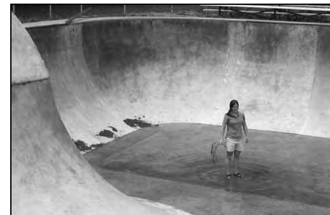
Water will render any skatepark unusable. Water should be carefully controlled throughout the skating area. On steel ramps, small holes can usually be drilled to prevent rust and drains should be kept clear.
